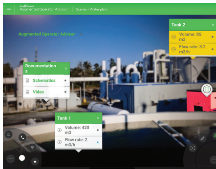
Outside the industrial site
