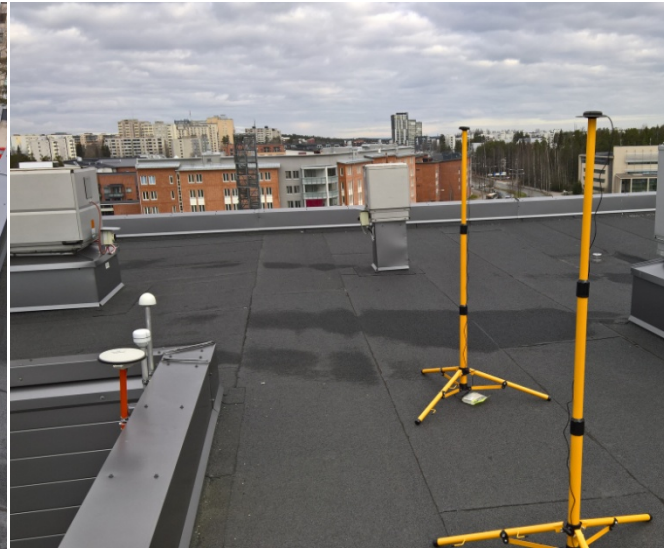
Base antennas 1, 2 and 3 looking north
