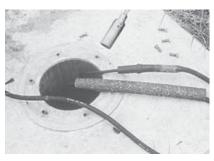
Pre-heat cable jacket. Begin shrinking at center, working toward both ends. Use a back-and-forth, sweeping motion of the torch.
