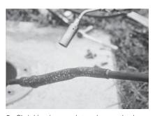
Shrinking is complete when melted sealant is squeezed from both ends of the sleeve and all heat-sensitive paint has changed from blue to gray.
