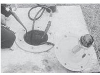
Slide the sleeve over cable before making electrical connection. Mate connector sections and wipe dirt from connector and cable. Clean cable with solvent wipe.
