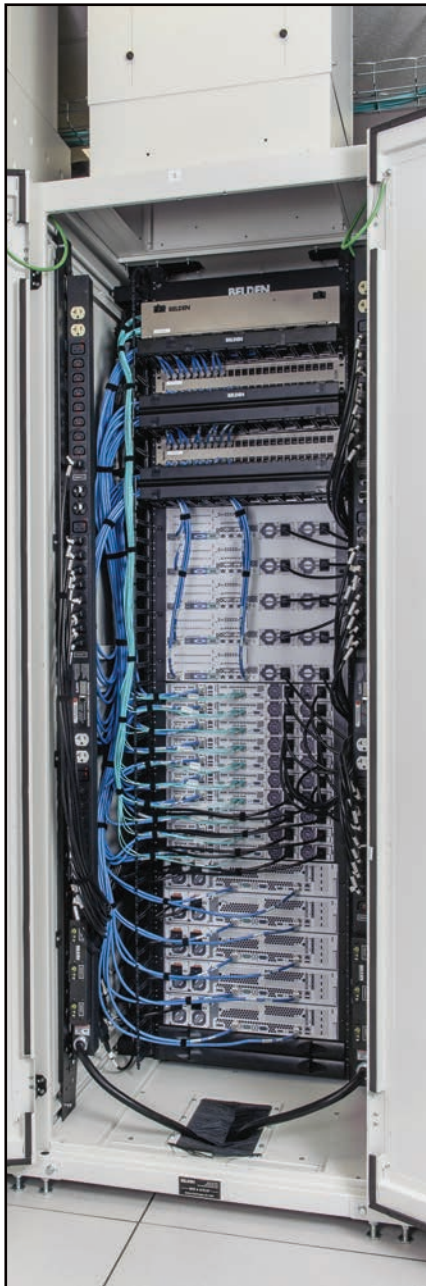
Side-by-side PDU mounting using 7" wide PDU mounting panel (Part No. HVMP024501)
