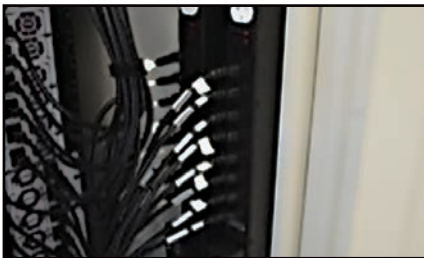
Side-by-side PDU mounting using 7" wide PDU mounting panel (Part No. HVMP024501)
