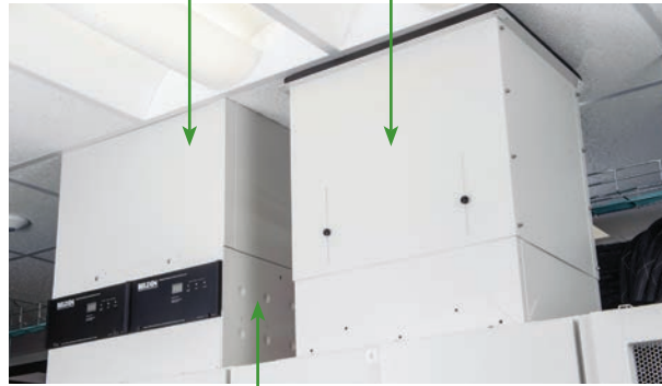
Example of passive and active chimney systems
