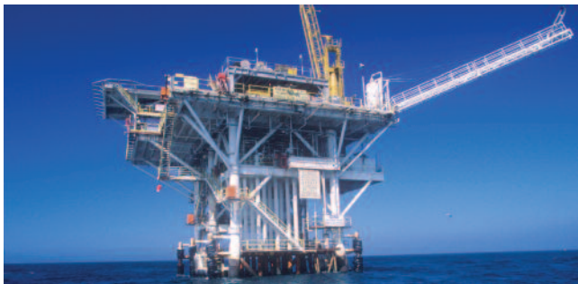
Offshore / Civil Marine
