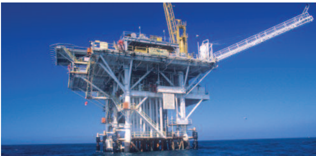
Offshore / Civil Marine
