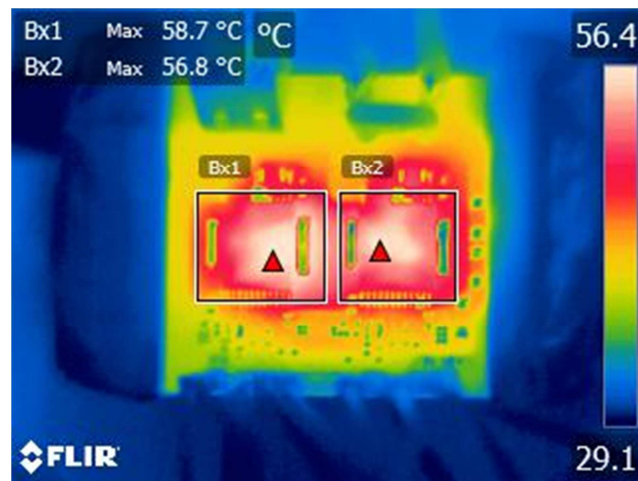
Figure 20 – Thermal Scan at 30 W Inverter Output in Self-Supply Operation.
